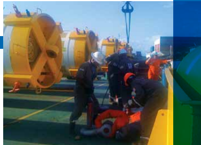
Suction-to-Stability (STS) heads are installed on the conductors.
